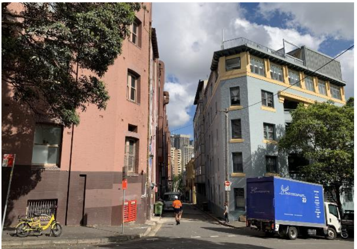
Figure 15: Looking north-west along Foley Street as viewed from Palmer Street, with Group 2 on the left and 265 Palmer Street on the right
