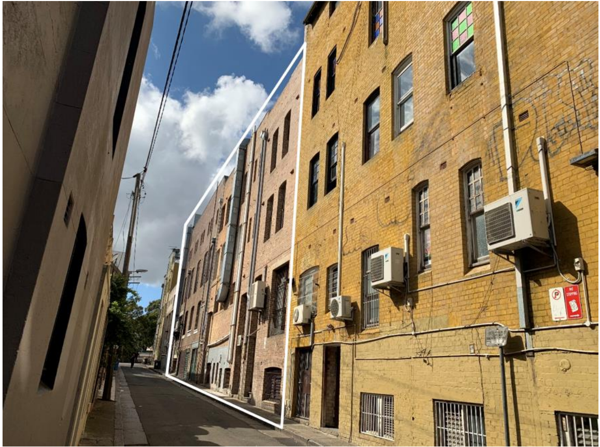
Figure 25: The site viewed from Foley Street
