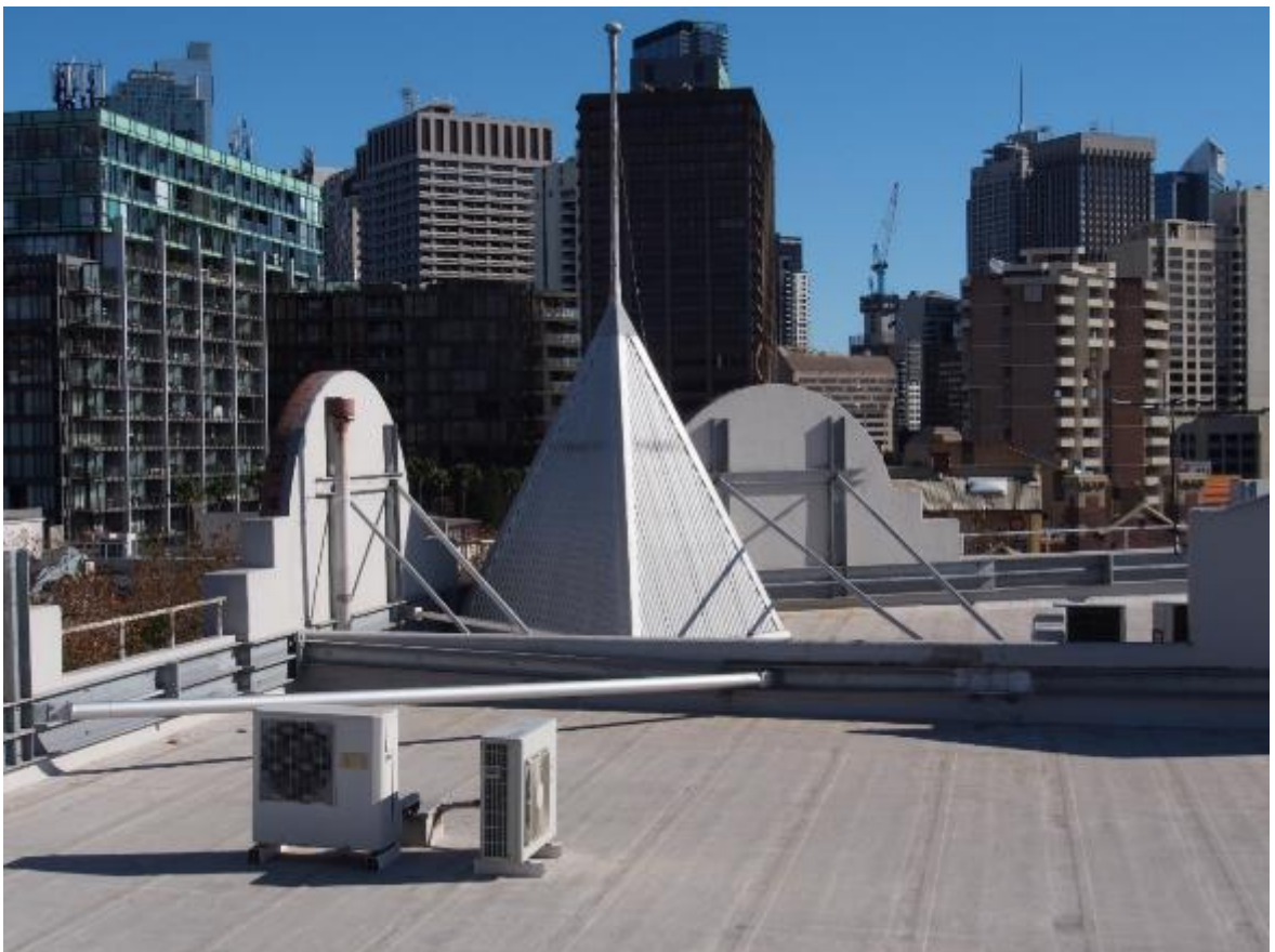
Figure 23: Feature pyramidal base to flagpole on Group 2 roof
