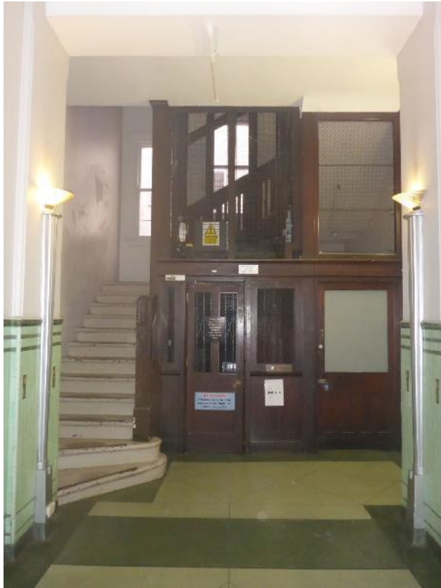
Figure 18: Original lift shaft and stairs of Group 2
