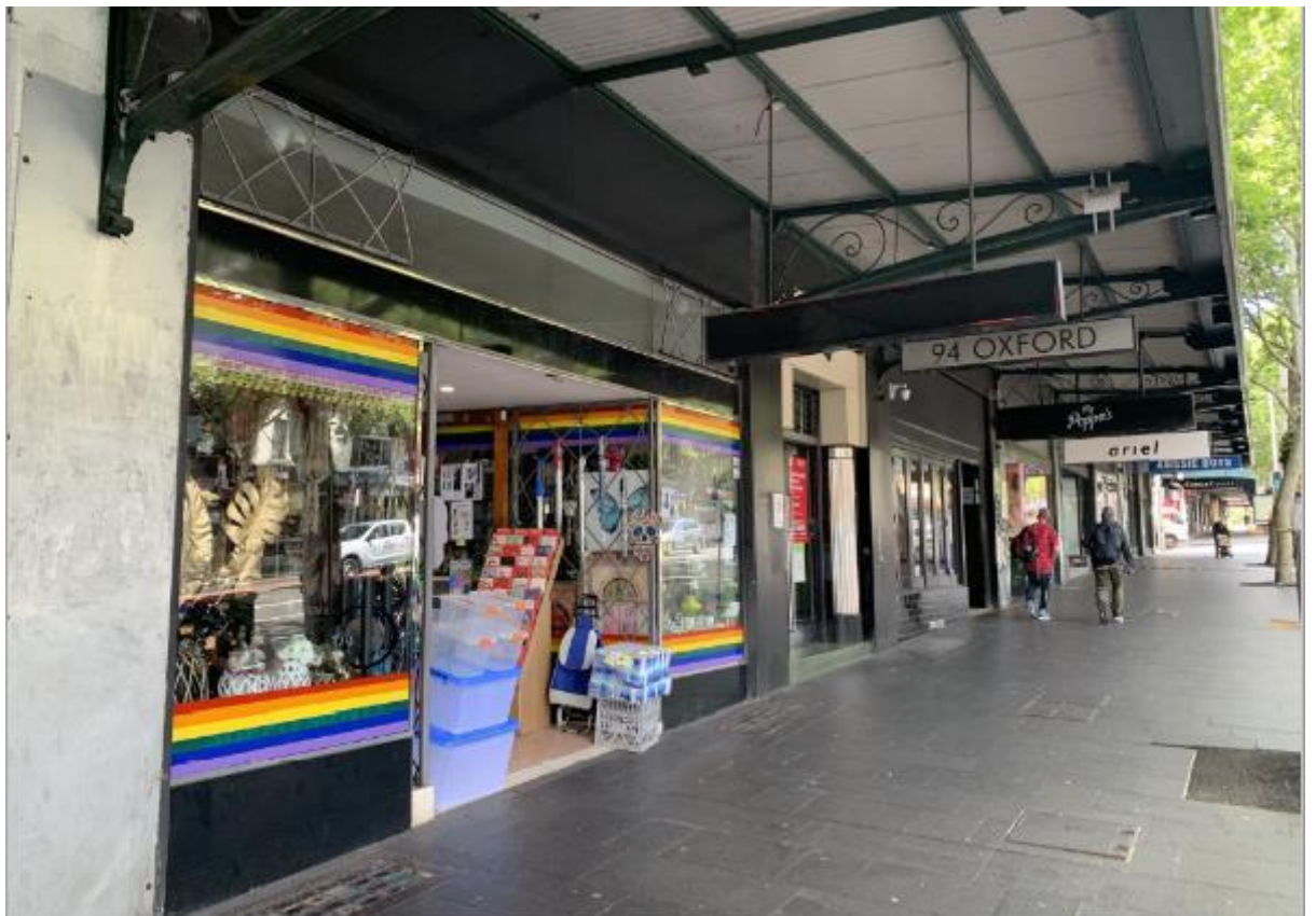
Figure 13: Shopfronts of Group 2
