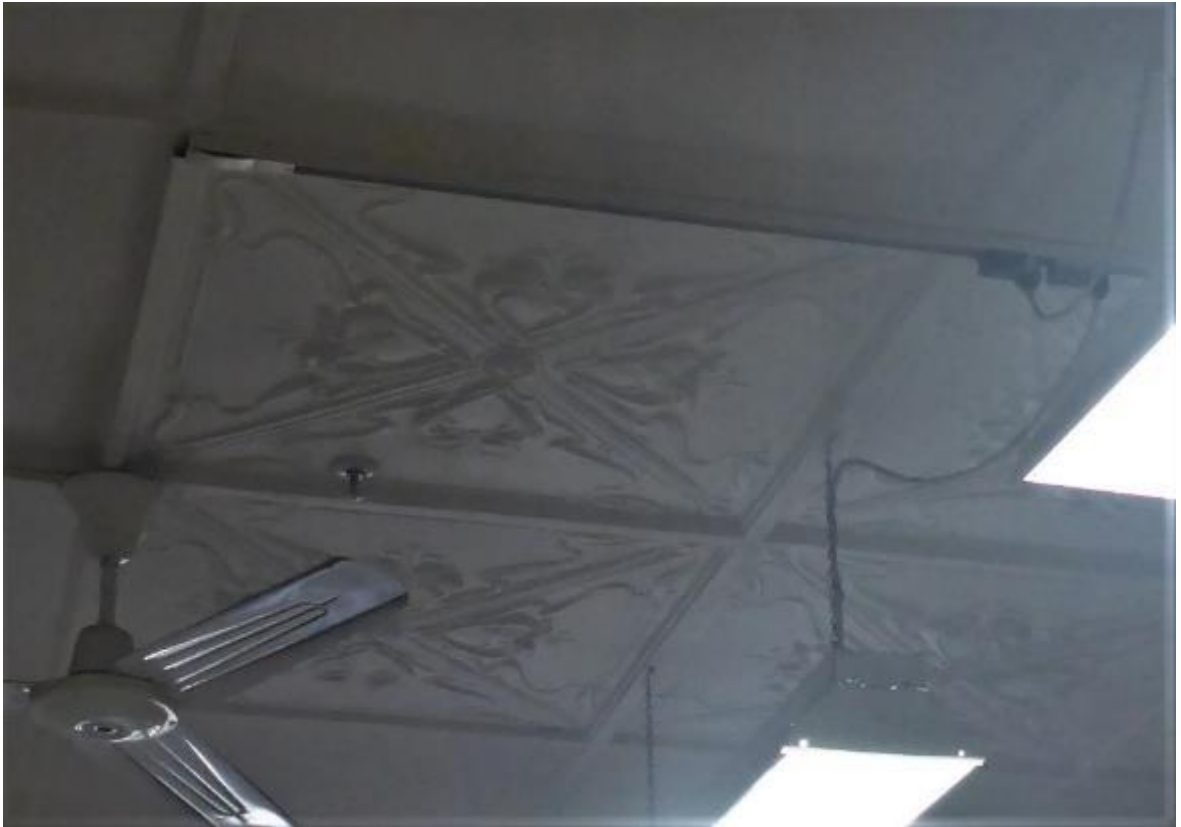
Figure 22: Original ceilings within Group 2
