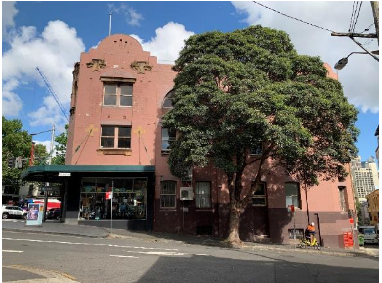
Figure 12: Group 2 as viewed from Palmer Street
